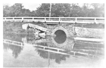
The stone arch bridge, reconstructed in 1931 when the roadway was concreted, only lasted for seven years. It was badly damaged in the 1938 hurricane and had to be replaced. Note the white fence railings. This view is probably of the south side of the bridge. The replacement bridge, finished in 1939, was of a more "modern" box culvert design, with stone railings. This 1939 bridge was reconstructed in 2013.
