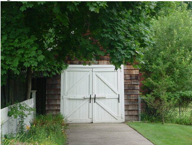
Figure 3 – Garage in rear (east) lot, west façade
