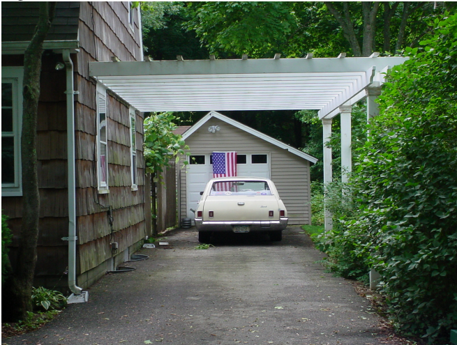
Figure 3 – Garage in rear (west) lot, east façade
