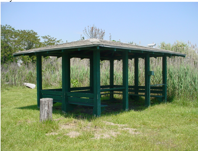
Figure 3 – Gazebo near the entrance, southwest elevation
